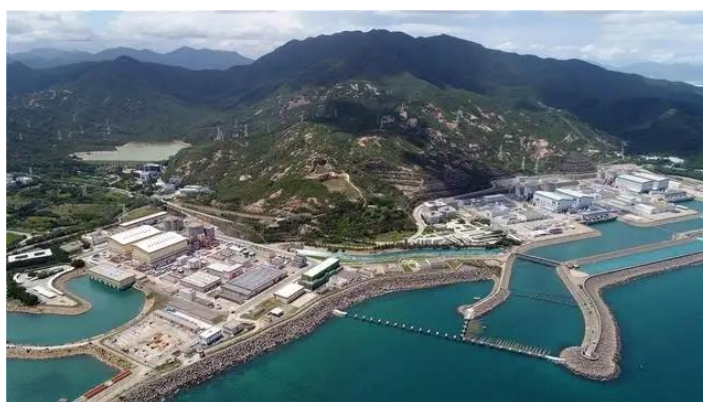
Figure 1 Lingao Nuclear Power Station of Daya Bay nuclear power base
