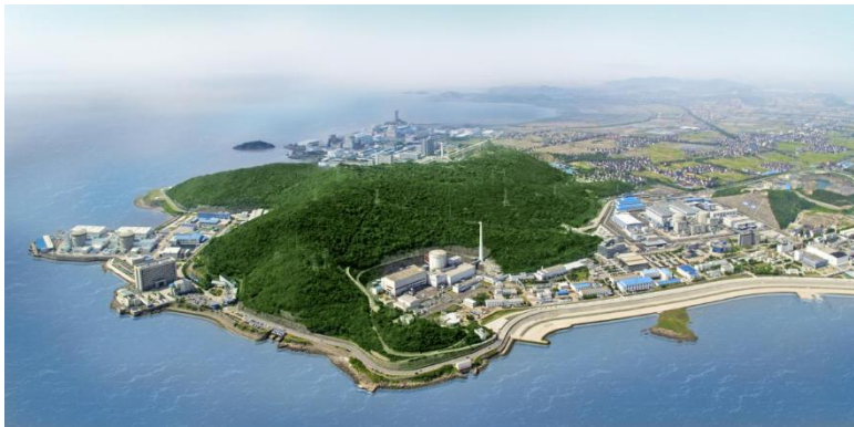
Figure 1 Qinshan nuclear power plant
