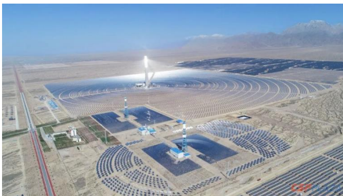
Figure 3 Aerial view of power station
