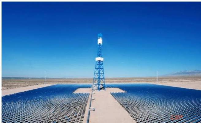
Figure 2 Close shot of the power station
