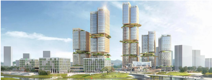
Figure 2 Shenzhen International Low Carbon City Cultural Conference Center
